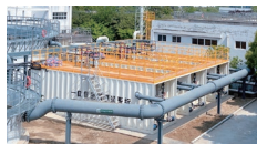
Skid-mounted (Capacity: 20-400 m 3 /h)
